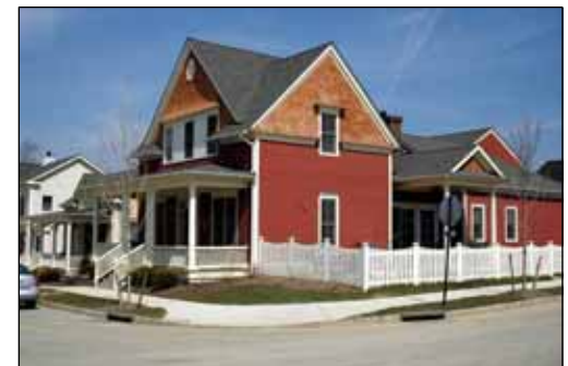
Upper Photo: Views of sidewalks along Route 9W.
